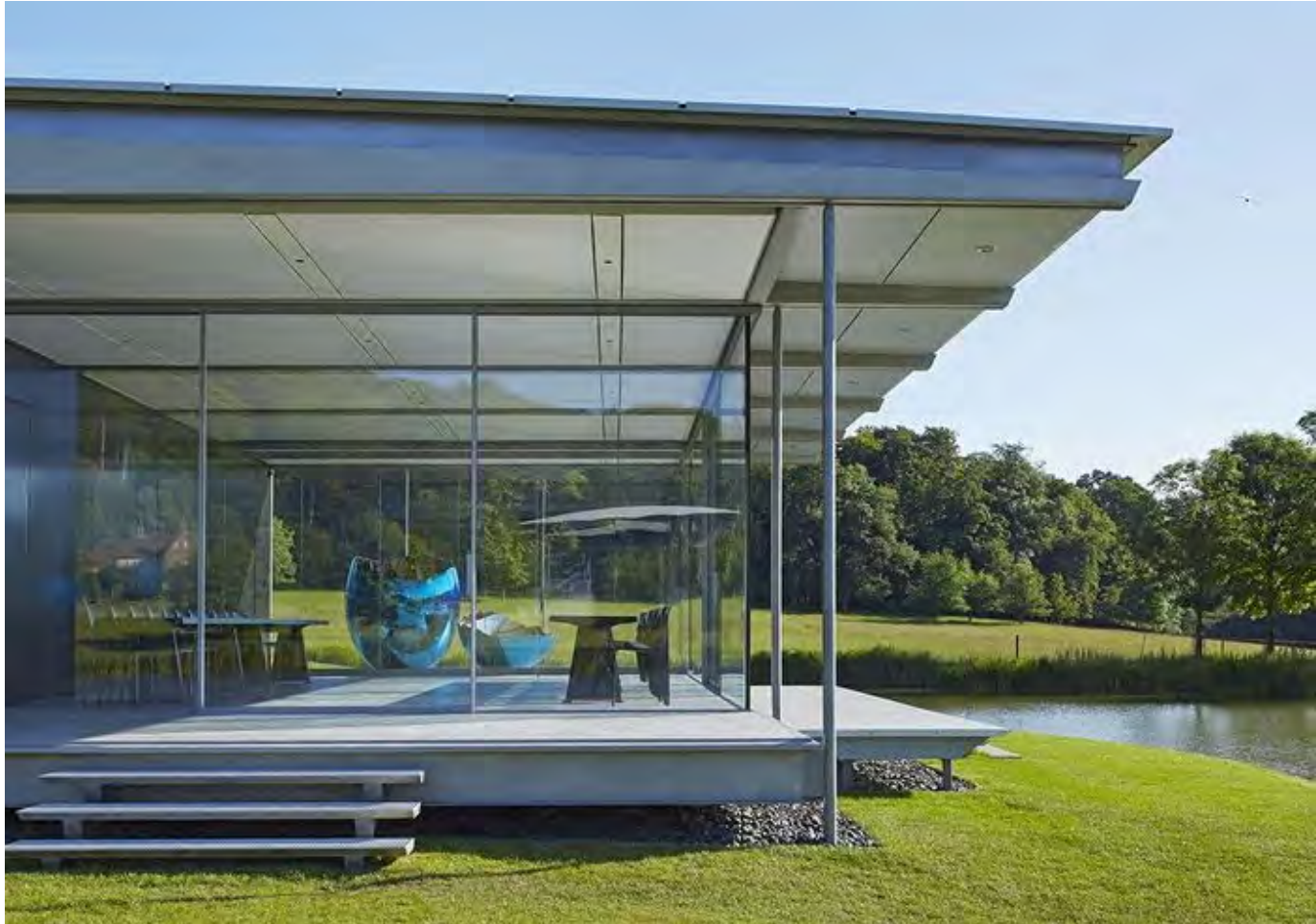
Island Pavilion and Footbridge, Wormsley – Architect: Robin Snell and Partners. Click on the image
