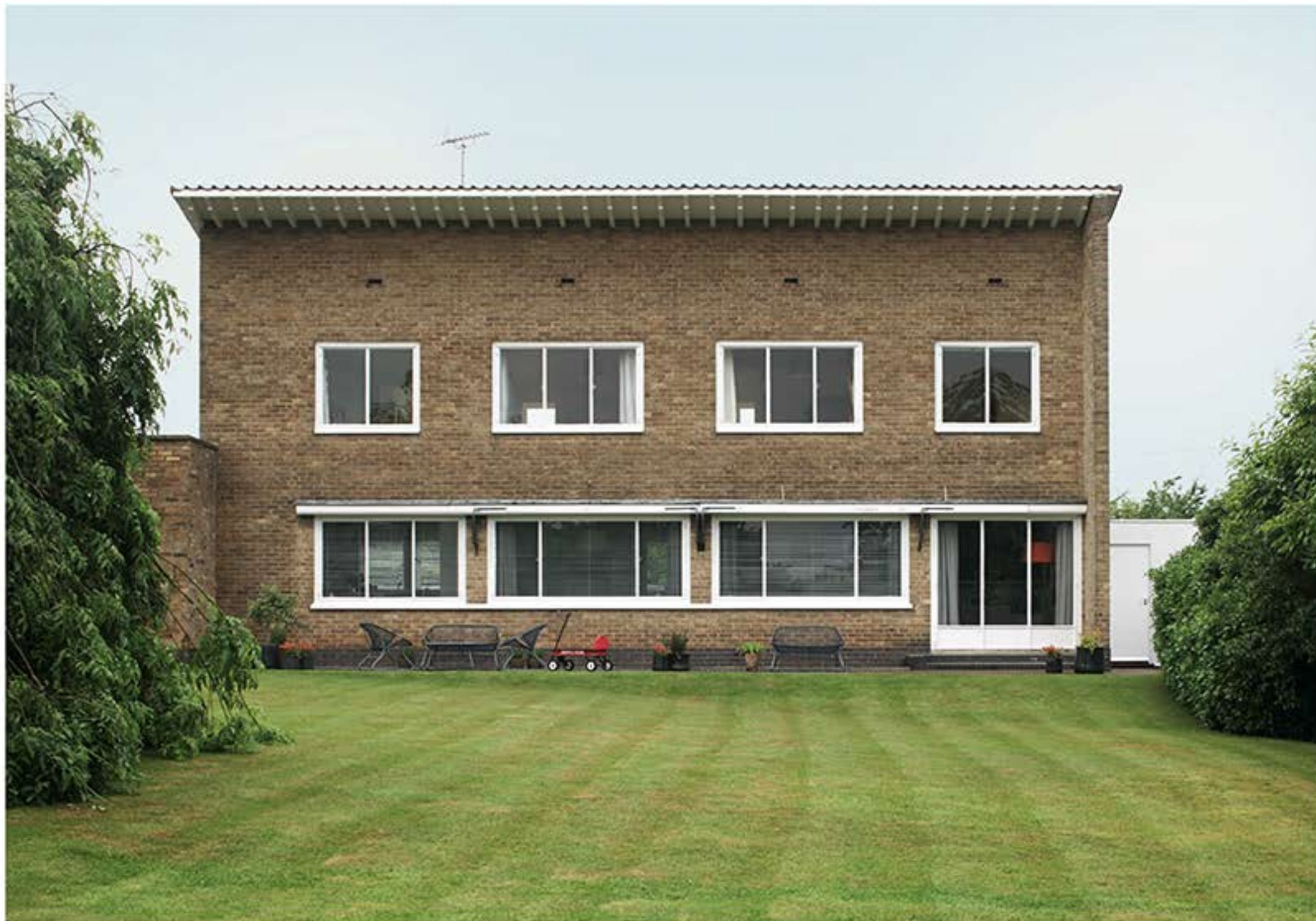
Above: external view from back.
